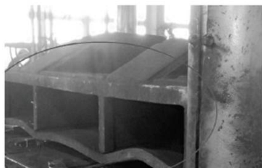
翻新前尾梁 Renovate the front tail beam
