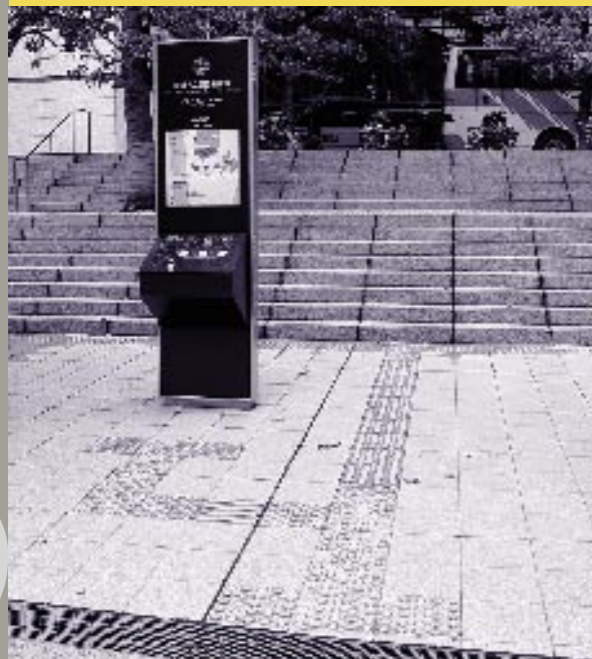
Position tiles in front of a signboard 指示牌前的方位引路磚瓦
