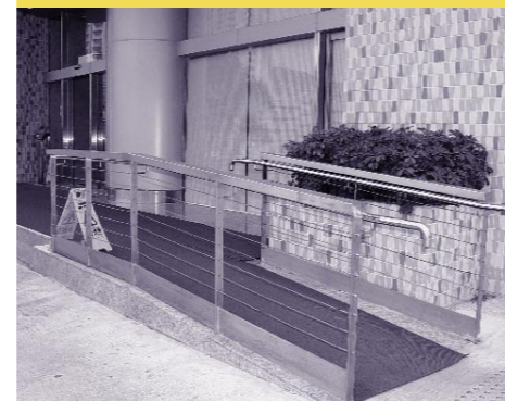
A ramp close to the building entrance 建築物入口的斜道
