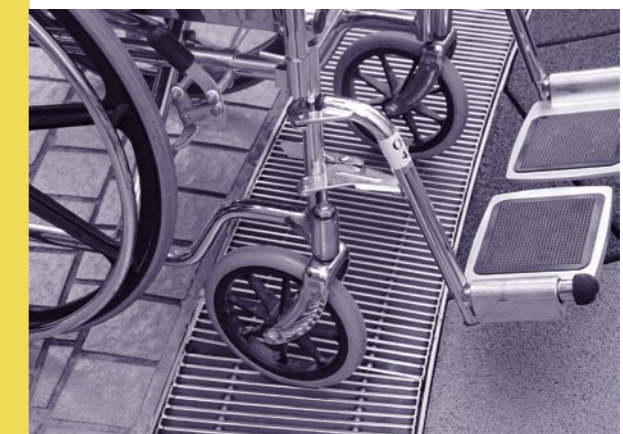
Preferred opening size of channel grating slots 渠道格柵的推薦開口尺寸
