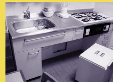
Knee space for the sink and stove 洗滌盆和爐具下的膝部空間
