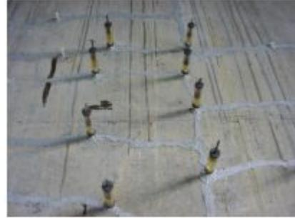
灌缝胶低压慢注裂缝修补工艺
