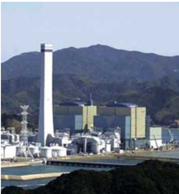
Fig. 2— Tachibana-Wan Thermal Power Station. The No. 2 unit is at right.
