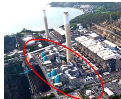
青山B廠脫硫除氮裝置項目 Castle Peak B Power Station EC Project
