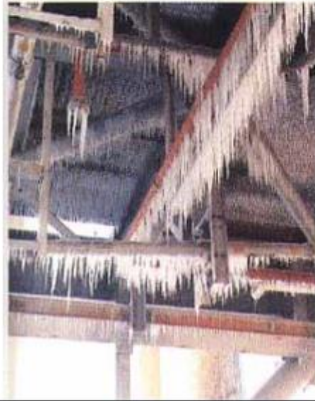
Above, foot long icicles on a lower level of the Fixed Service Structure frame the attachment point where the Orbiter is attached to the external tank (arrow). Icing was even more extensive all upper levels of the service structure (upper right and below). At right below is a ground communications box (not used during launch) rendered inoperable by heavy ice.
