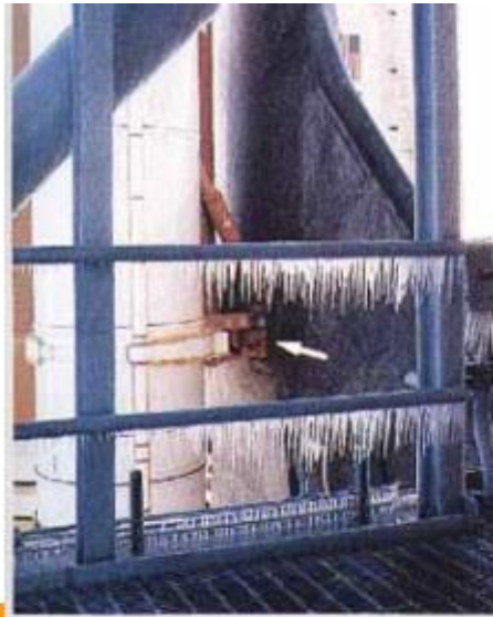
Above, foot long icicles on a lower level of the Fixed Service Structure frame the attachment point where the Orbiter is attached to the external tank (arrow). Icing was even more extensive all upper levels of the service structure (upper right and below). At right below is a ground communications box (not used during launch) rendered inoperable by heavy ice.
